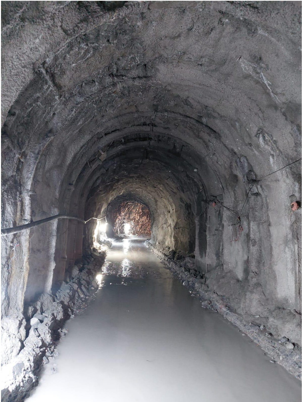
Figure 16: Gravel Flushing Tunnel
