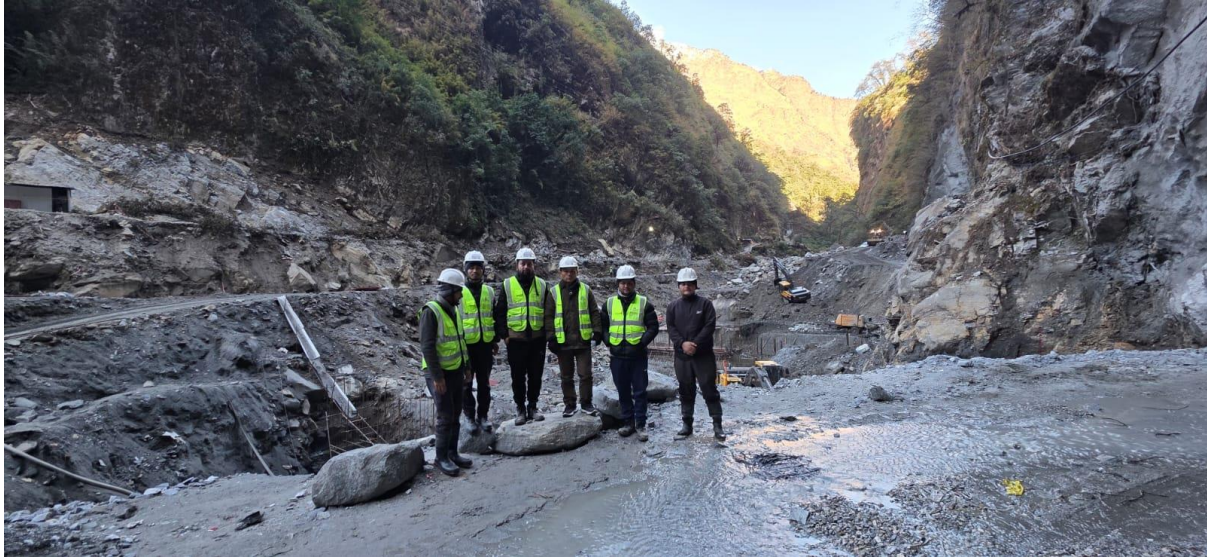
Figure 21: High Levels on Site Inspection
