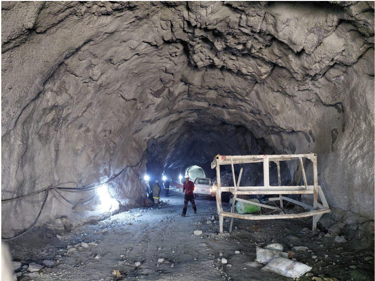
Figure 15: Gravel Trap Tunnel
