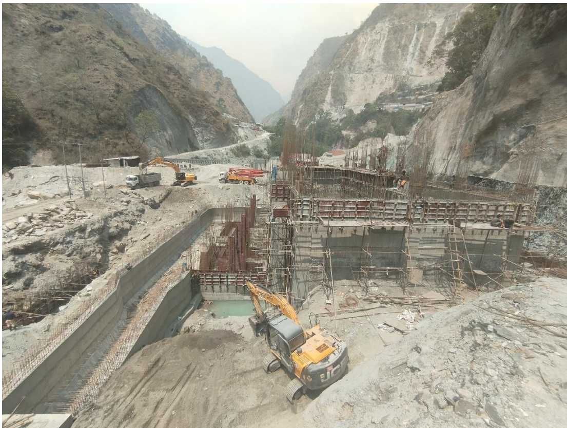
Figure 25: Completion of Powerhouse Upto Loading bay Level
