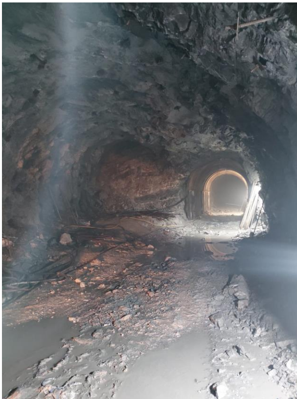
Figure 10: Desander excavation going on
