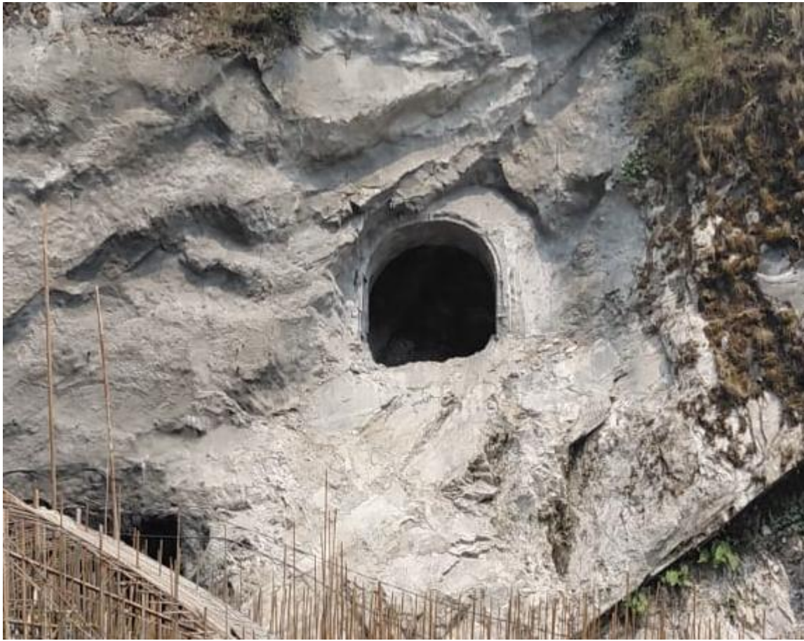
Figure 14: Undersluice Platform tunnel portal
