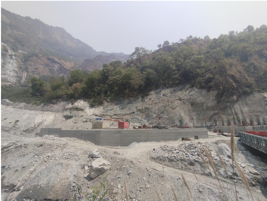
Figure 24: River protection wall on Powerhouse
