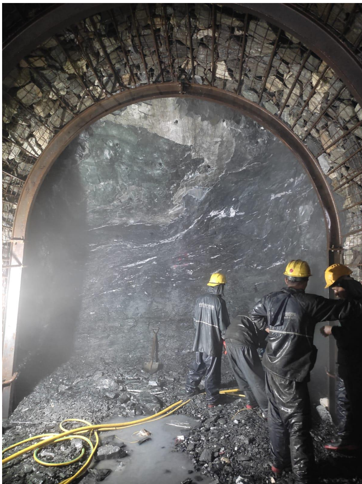
Figure 18: Adit 4 HRT outlet
