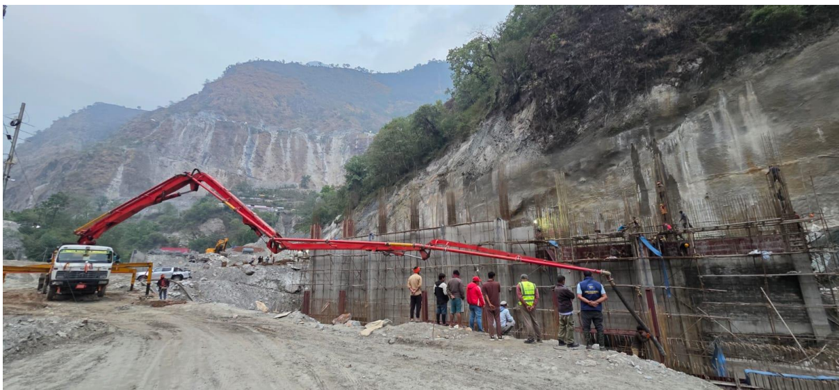
Figure 22: Concreting works on powerhouse
