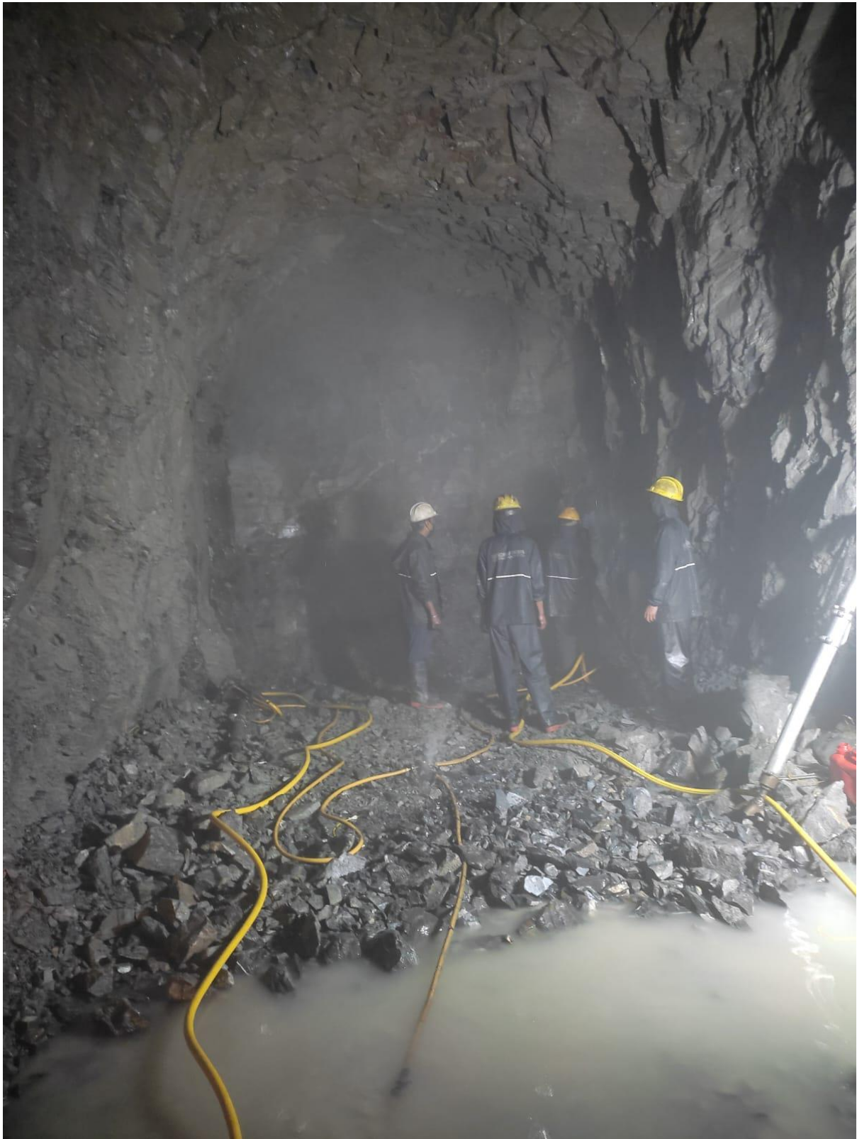
Figure 17: Adit 3 HRT US Tunnel
