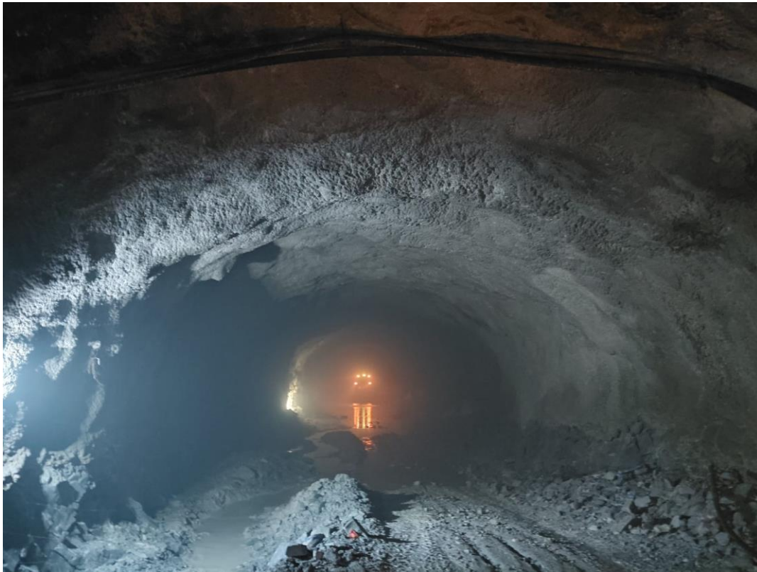
Figure 9: Desander excavation going on
