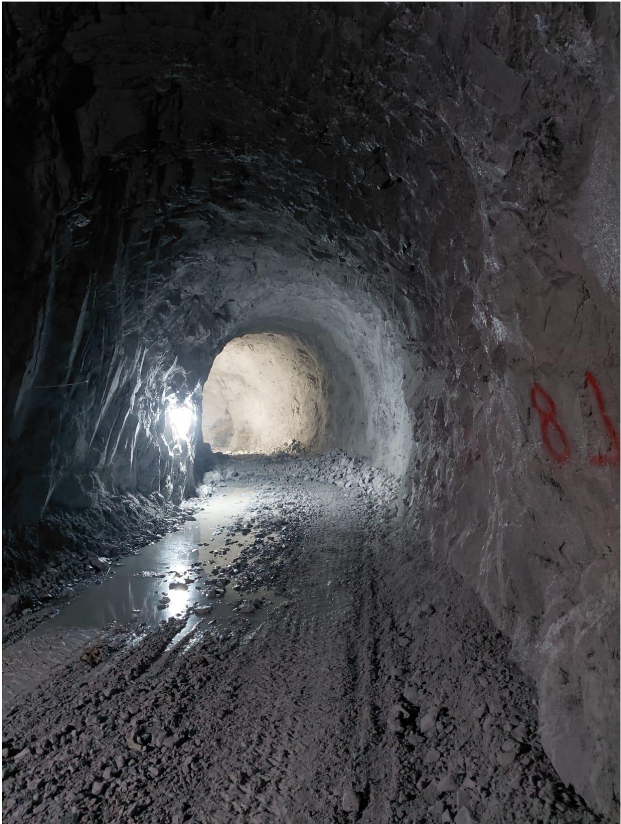
Figure 12: Gravel trap operating tunnel
